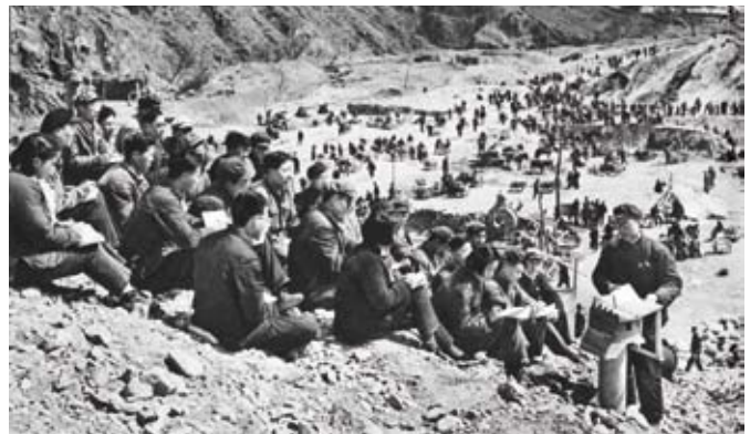
A field study class held at the construction site of Miyun Reservoir
